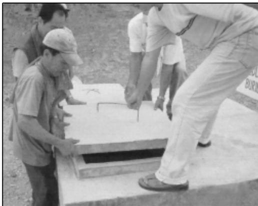
Photograph 18. Cover of a Rectangular Concrete Septic Vault
