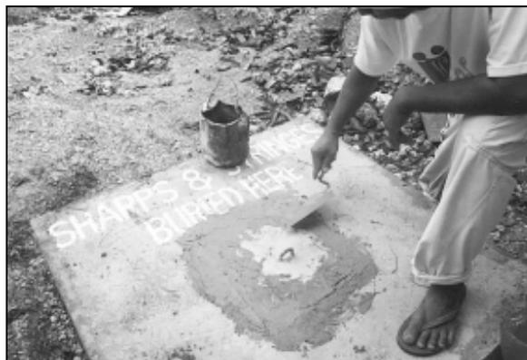
Photograph 23. Sealing of a Concrete Vault
